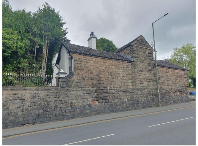
8. The outbuildings of the big house Rockcliffe, on Leek Road
