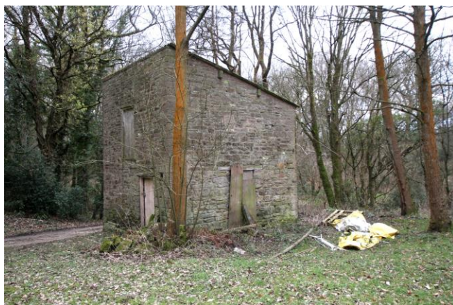
The building as it stands today. As can be seen the building has had quite a lot of height removed; this includes the part of the bob wall where the beam was situated. The shaft is located to the left of the bags with the spillway out of shot to the right
