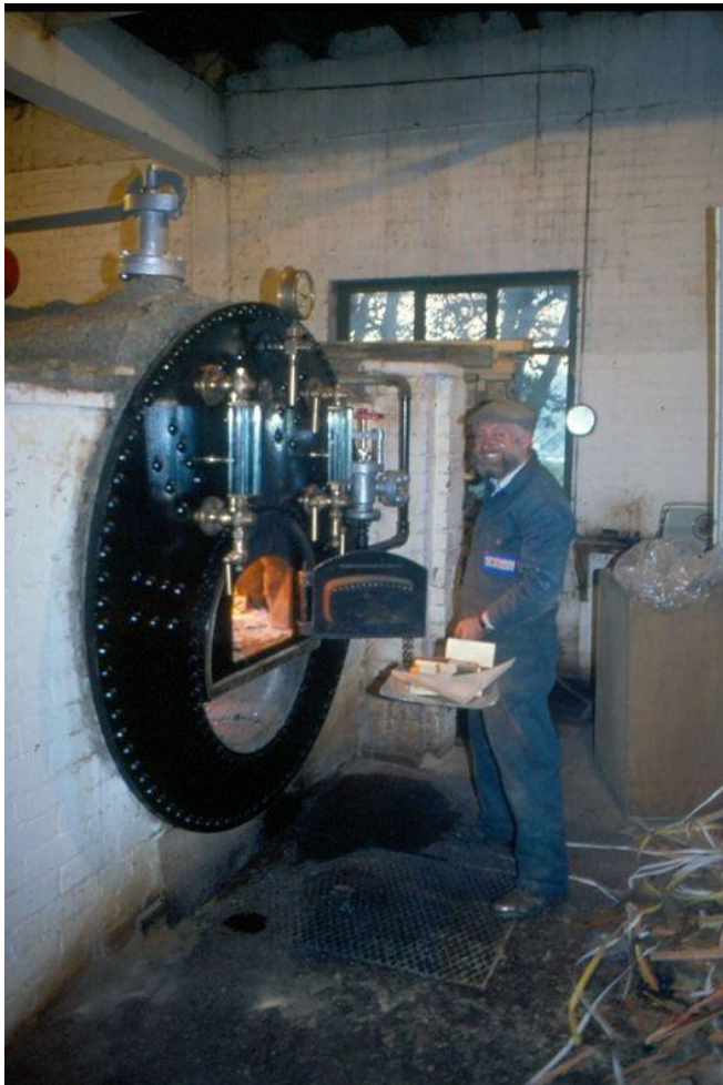
Lambert's Cornish boiler during a general overhaul around 1989. Photo Alan McEwen
