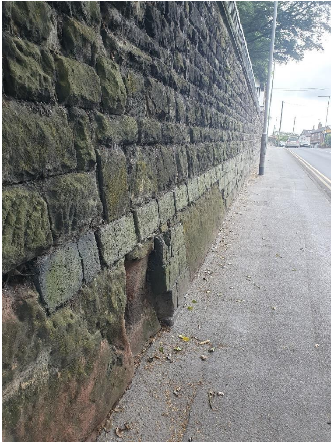
6. Looking north up Butler's Hill on Leek Road, Cheadle (A522), bedrock gives way to four courses of slag blocks, with several courses of masonry above
