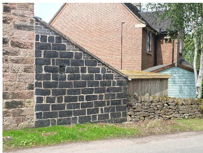
4. The single-storey lean-to extension at the north end of Bridge House
