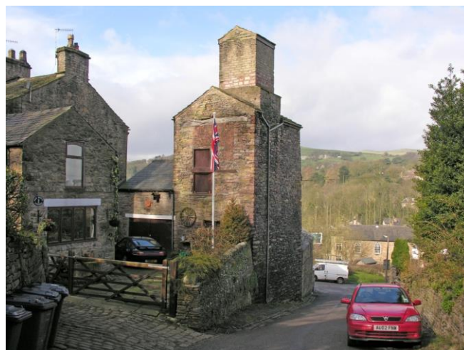
The Waterloo Pit Engine House as it is today
