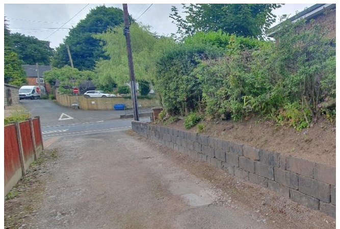
9. Opposite Rockcliffe, an un-named track leads east to a spot named on the map as Windy Arbour. The wall on the north side of the track is composed of slag blocks for a short way
