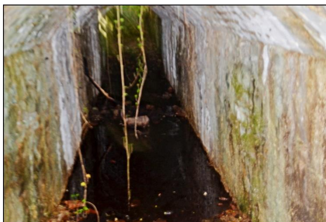
Relying on electronic flash to penetrate the gloom, a passage is revealed that runs below the units of the powder mill
