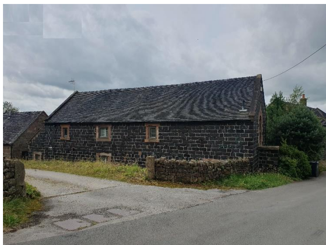
3. This building too has been converted to residential use and is now known as Shires Barn.
