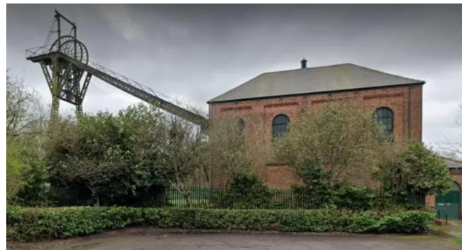
The F-Pit Engine House and the attached headgear are a Scheduled Ancient Monument and the only surviving structures of New Washington Colliery, which closed in 1968
