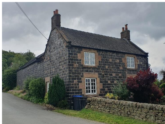
1. Stable House, and beyond it a building now converted to residential use and named Coach House
