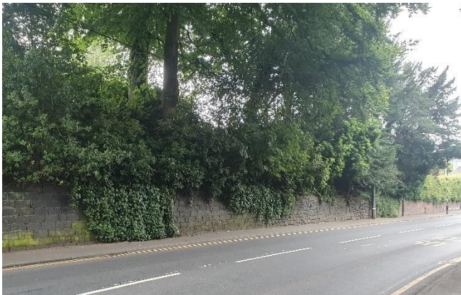
7. Opposite photo 6, the revetment on the east side of Butler's Hill on Leek Road is part slag block, part masonry
