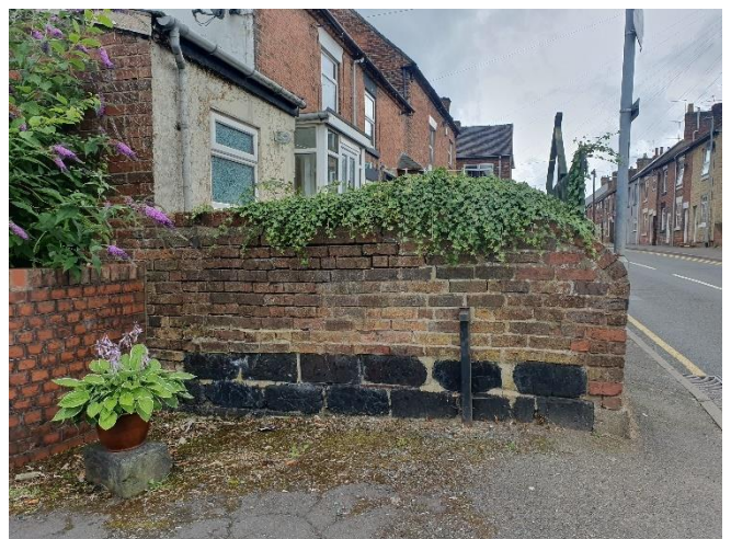
10. At No.90 Queen Street (B5417) a few blocks have been used at the foot of a brick wall. I would imagine these may have been recycled from elsewhere
