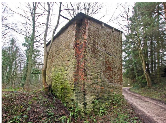
As it stands today showing location of the chimney with the entry for the cylinder on right side wall
