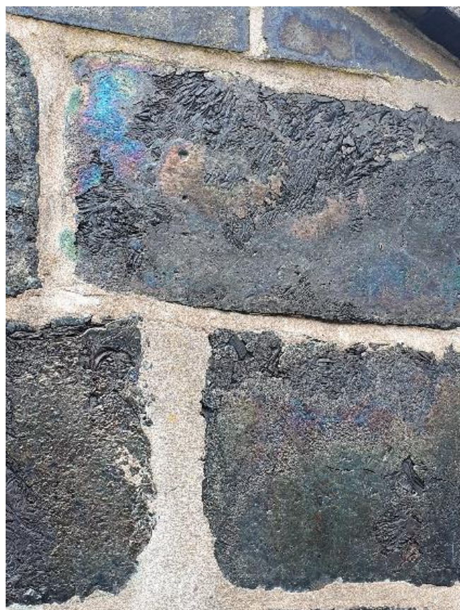
5. Close-up of the blocks at the Bridge House extension
