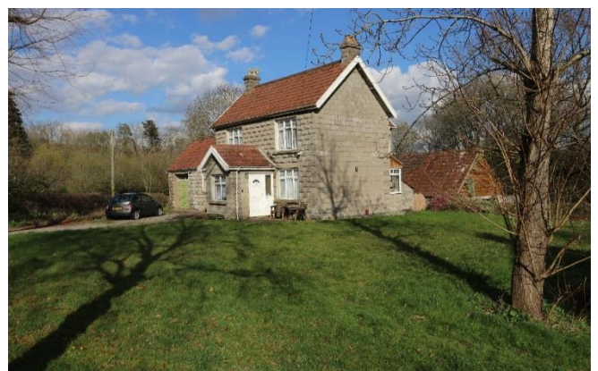
Plate 5 – No.108 Badminton Road, built by Mr Rodman in the interwar period and now owned by the Talbot Family
