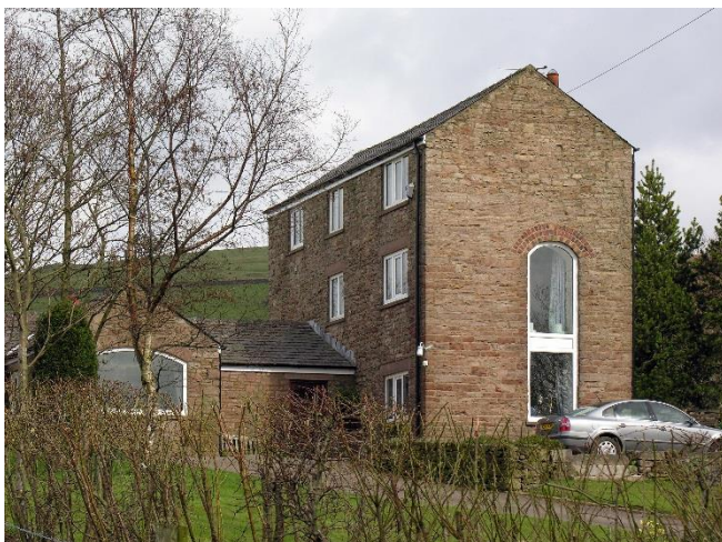
The house as it stands today. The boiler once stood at the left side of the main building with a chimney behind
