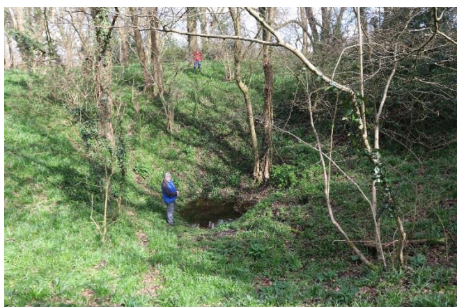
Plate 7 - The largest hole in the brake via which Mr Rodman's coal workings were reportedly accessed
