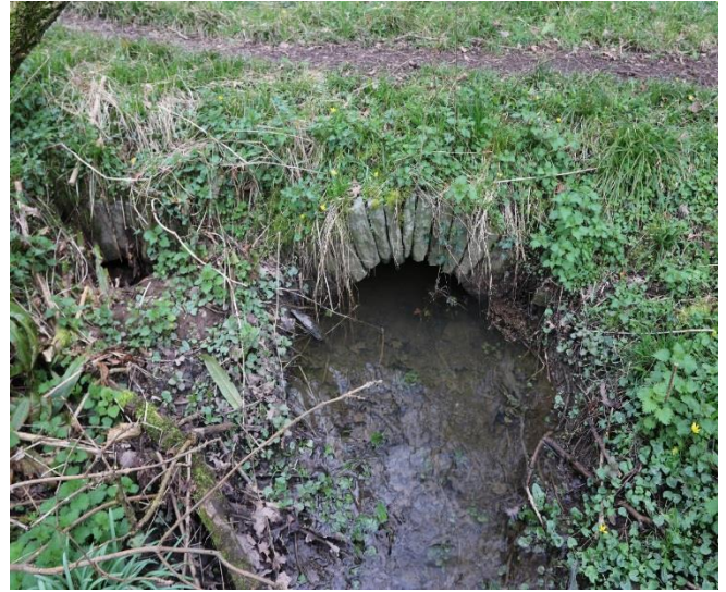
Plate 2 – The twin arches of the bridge appear to be built using the local pennant stone. The bridge may be of a considerable age (one arch shown in photo)
