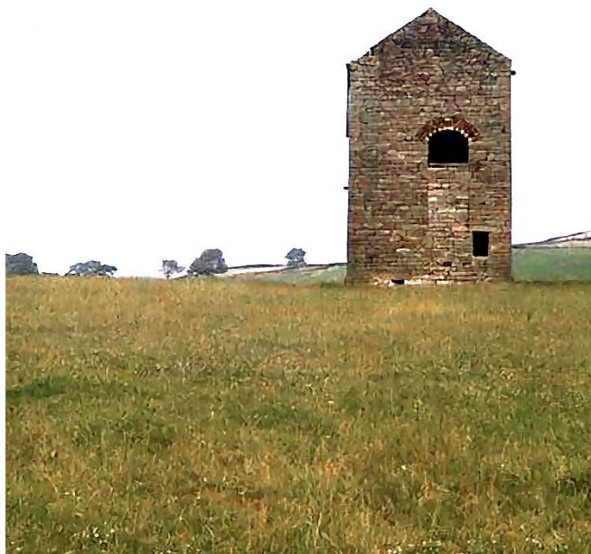
The building housed a rotative beam engine used for winding coal from the shaft, which was located between the camera and the building (Photo 1975)
