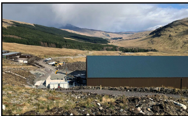
Processing shed: The Cononish mine building that now graces the West Highland Way
