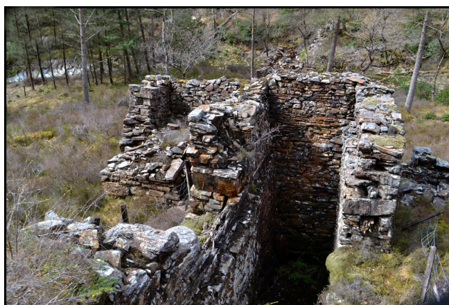
Fig 02 The pit of the waterwheel. Note the river Mawddach, top left
