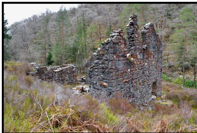
Fig 01 First view of the processing mill, previously concealed by trees and vegetation
