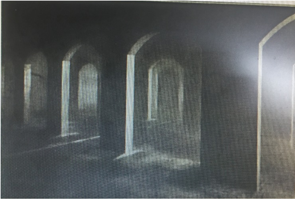
The underground Res made of concrete with metal rebar.
