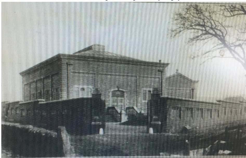
The main building where the pumping engines were installed. The smaller one is the workshop and other areas.
